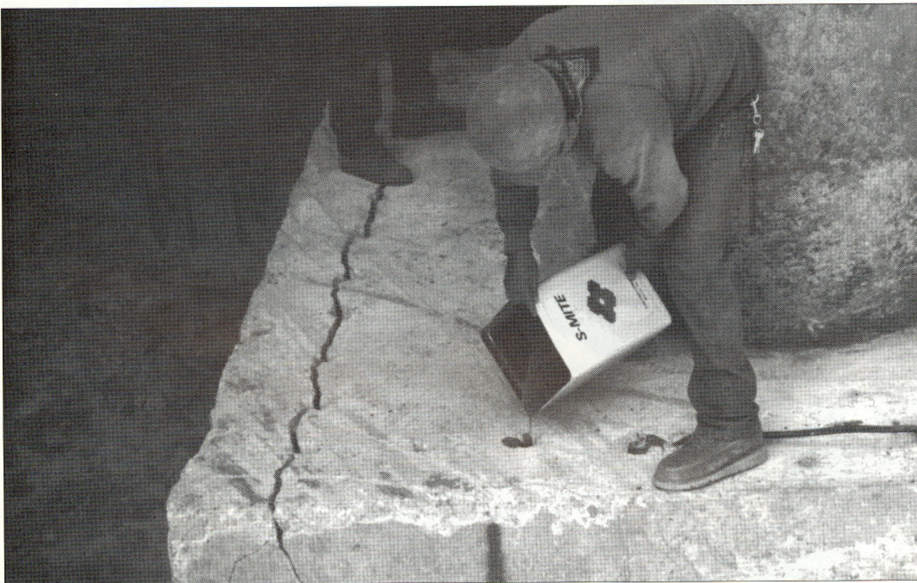
S-Mite is poured into drilled holes along one side of the footing. The crack along the left side of the footing shows the results of the S-Mite after roughly 24 hours of expansion. The crack provides access so a backhoe bucket tooth can pull away the section.
